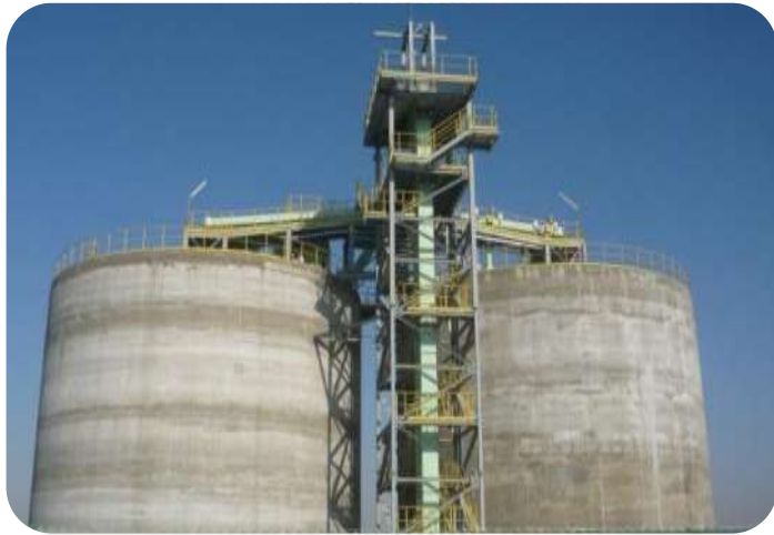
Product transport to cement silos
