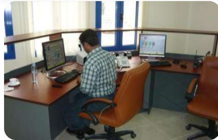
„Control room“ with visualisation
