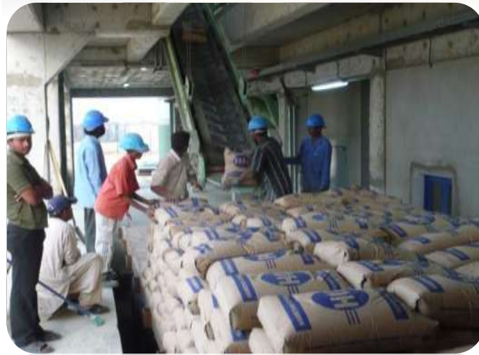
Loading of cement bags
