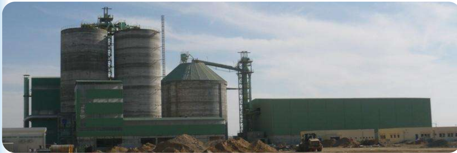
Grinding plant with raw material storage, clinker silo, mill building, cement silos & packing plant
