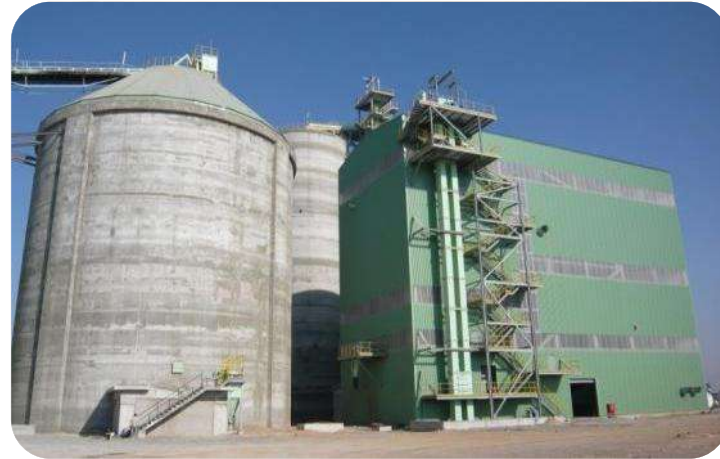
Clinker silo & infeed
