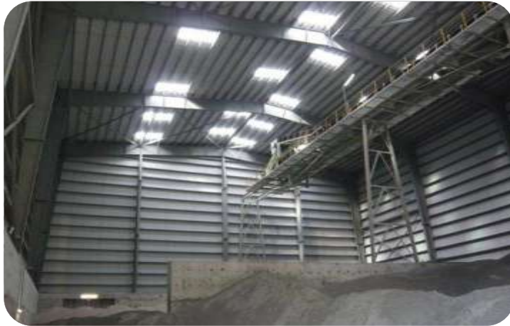
Raw material storage with „tripper car“
