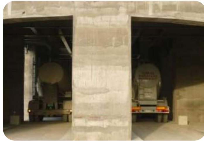
Loading of cement
