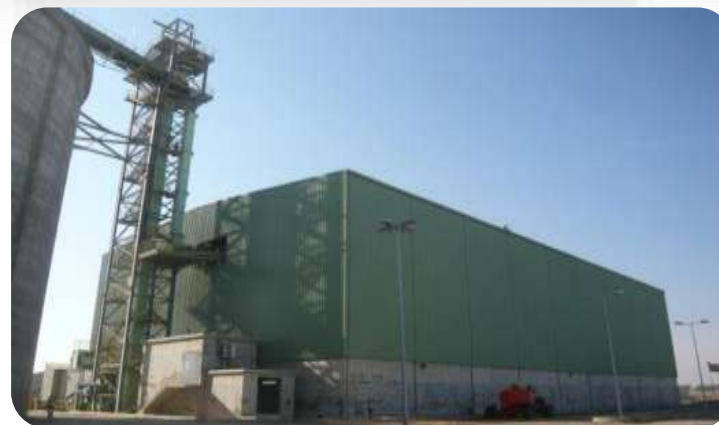
Raw material storage, feed via bucket elevator
