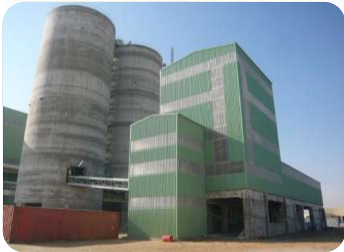
Cement silos & packing plant
